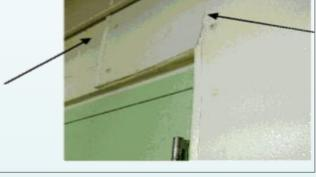
A coved juncture between floors and walls prevents accumulation of dirt
